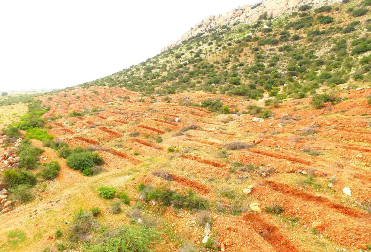
Staggered contour trench
