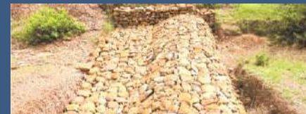
Construction of check dam
