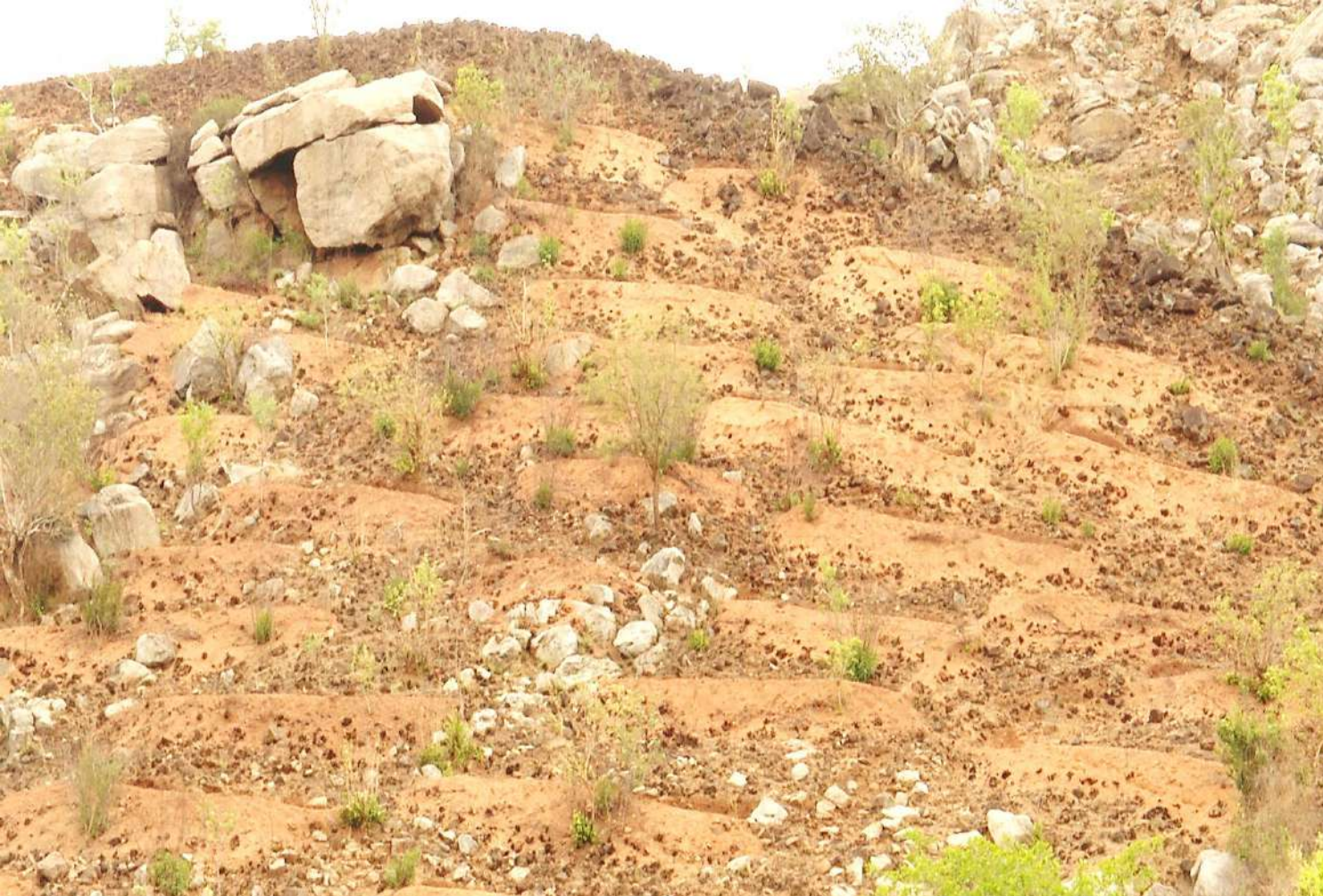
Staggered trenches on a hill
