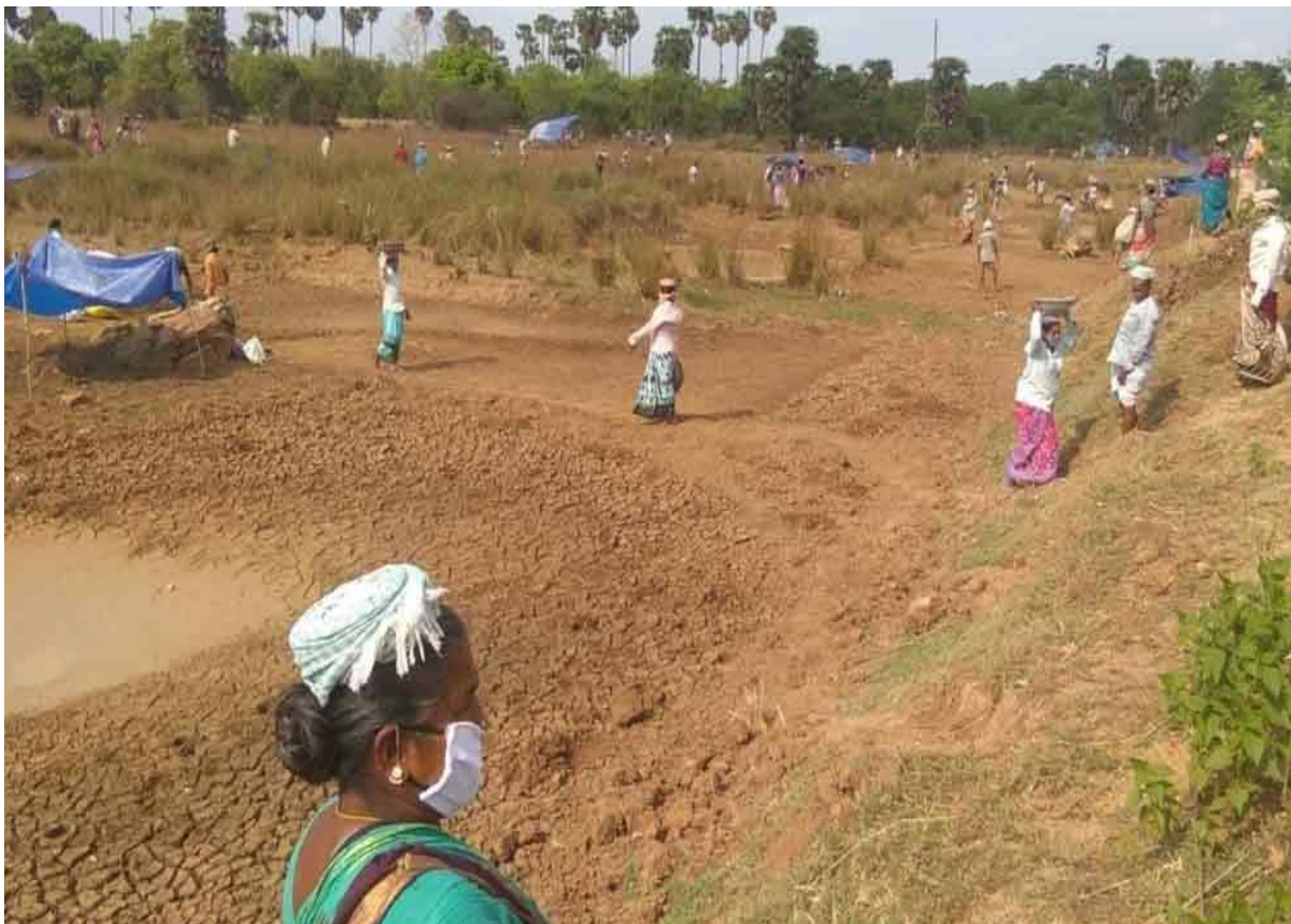
Figure 3: Workers during NAREGA works in Vizianagaram. (Photo | EPS)
